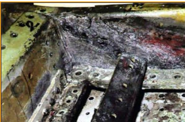
**Corrosion of: Damaged PRIMARY Protective Coatings**
